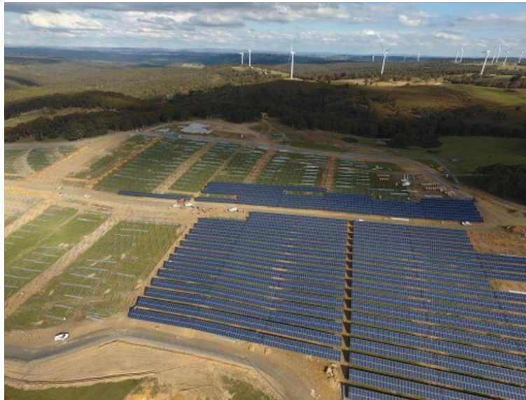
Photo: Gullen Solar Farm in advanced stage of construction.
